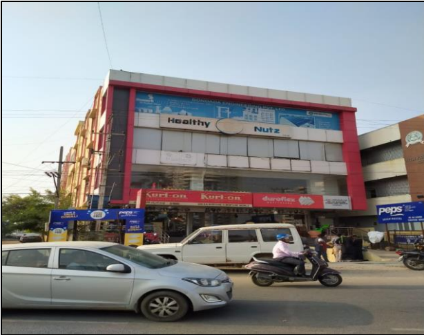
Outer view of the facility - I
